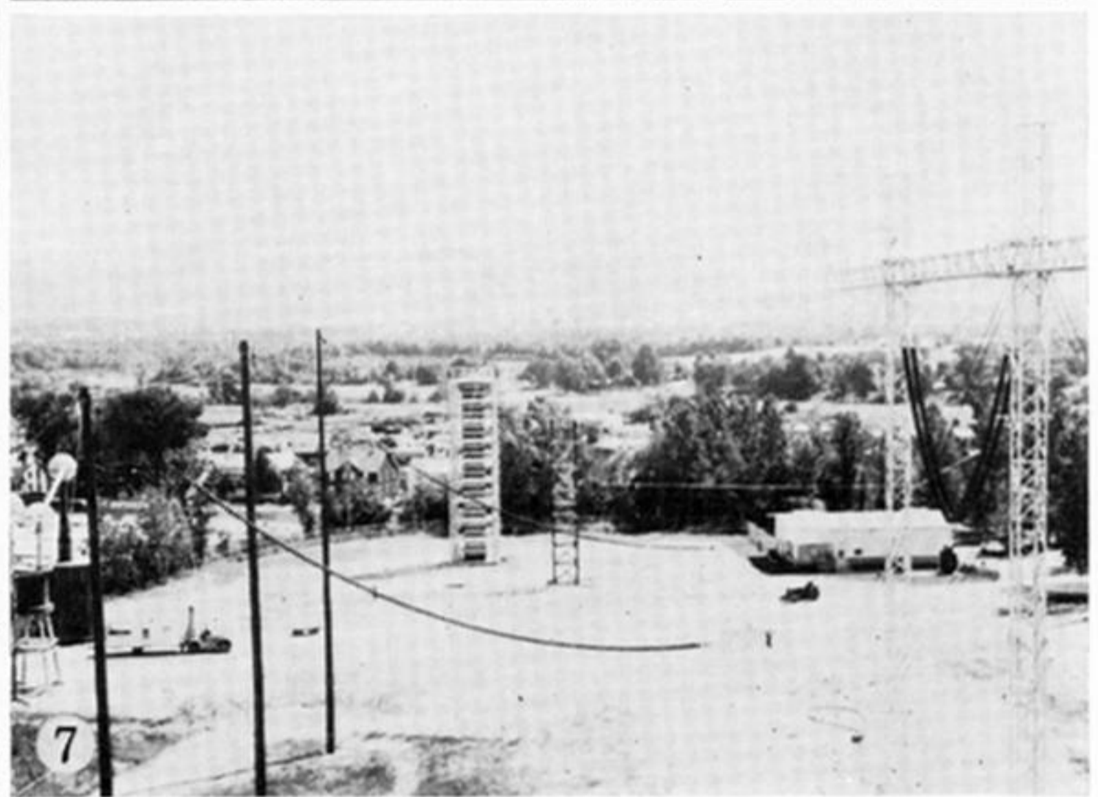
FIGURE 2. A view of Project UHV – a 1000 to 1500 kV transmission research project in Pittsfield, Massachusetts.
